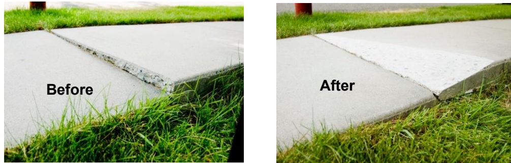
Figure 7: Precision Sidewalk Safety Work Example
